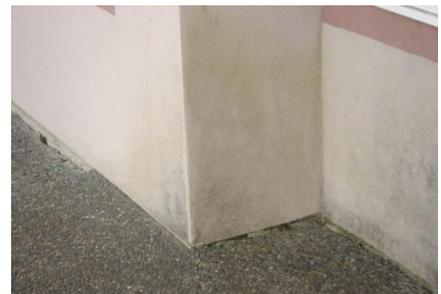
Figure 2 wet wall caused by negative slope
